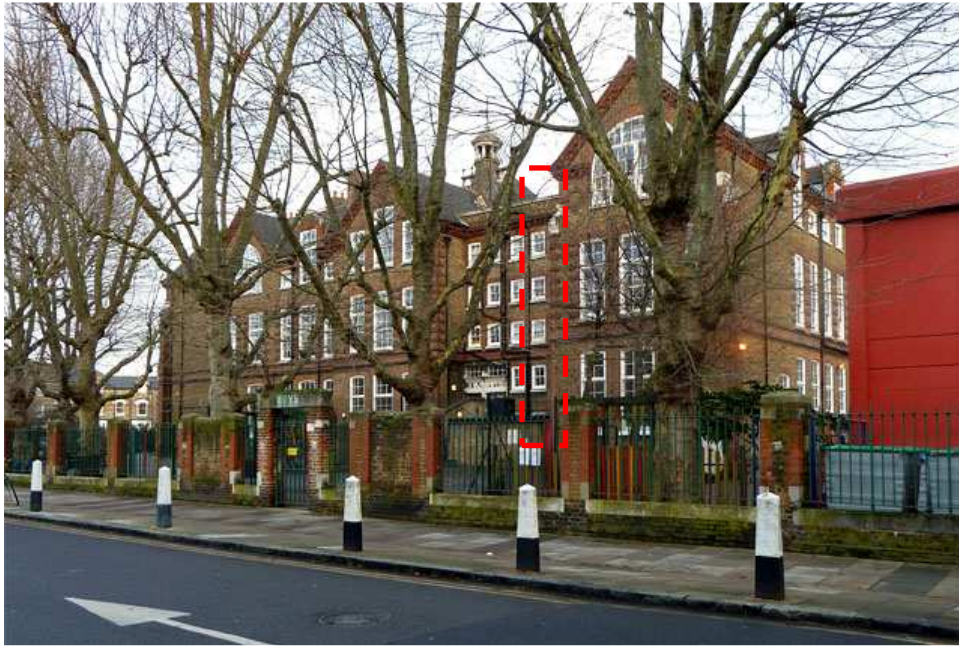
View from Perth Road Location of flue set behind decorative quoin detail
